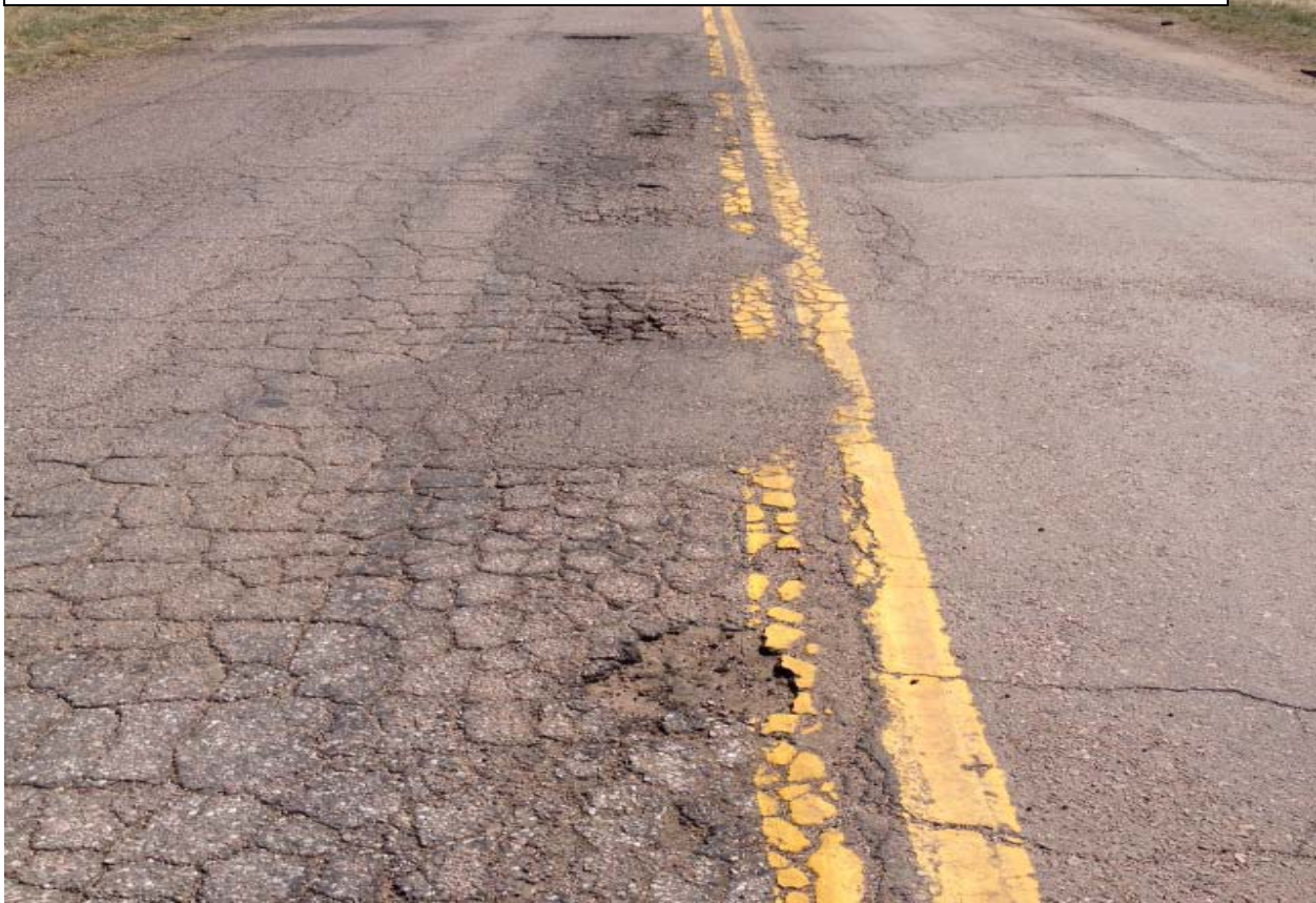
Picture 1: Charter Oak Ranch Road Degradation and Lack of Drainage Facilities
